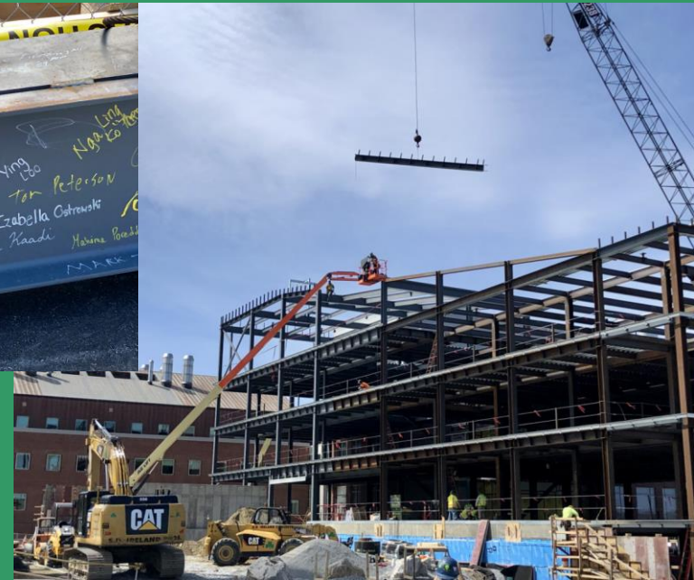
Topping Off & Beam Signing: 4/27/21
